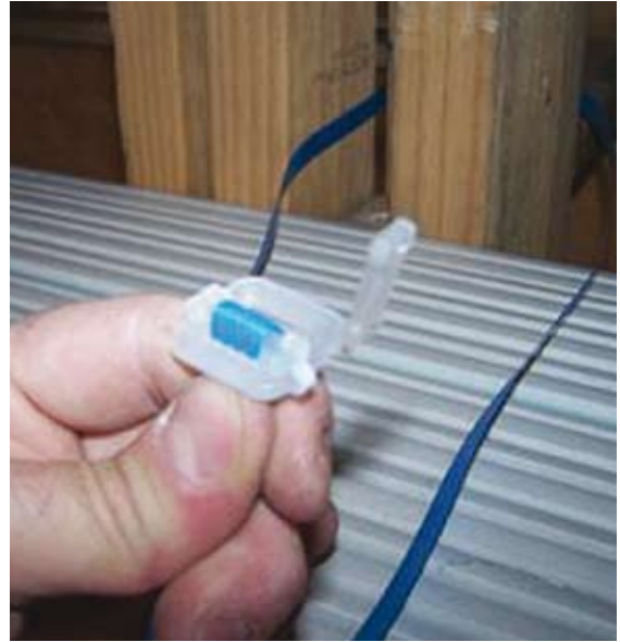
Example of edge stacked plasterboard secured by Poly Propylene strapping and buckle.
