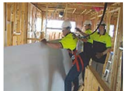
Example showing the use of a fall arrest harness
